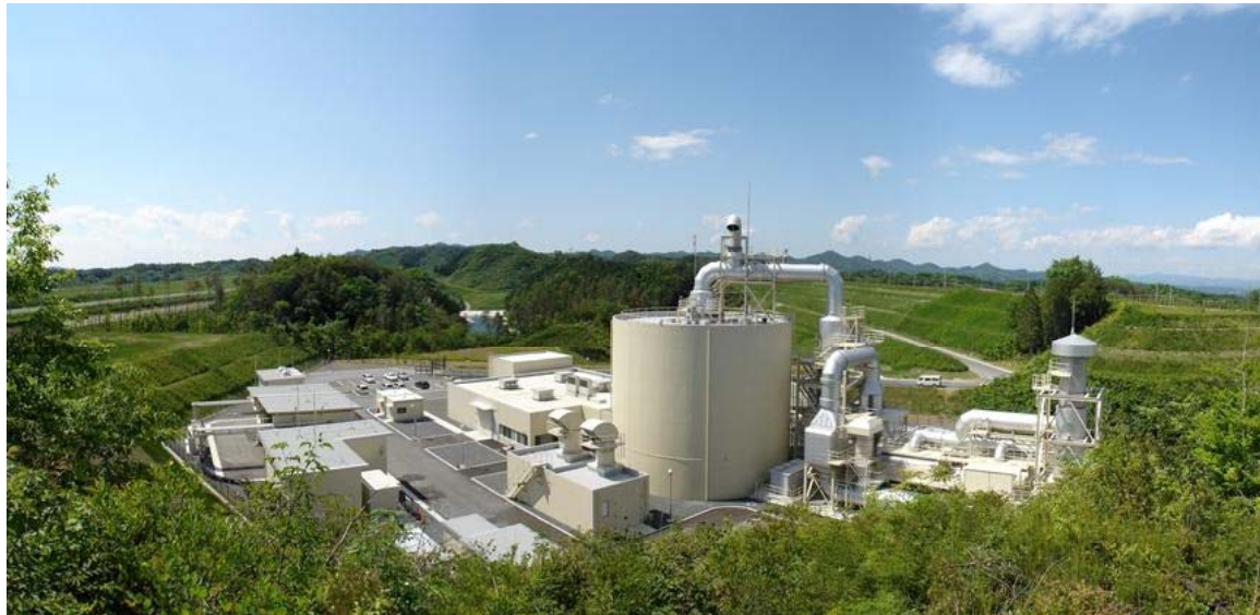
Hydrogen and Fuel Cell Vehicle Safety Evaluation Test Facility (Hy-SEF)
